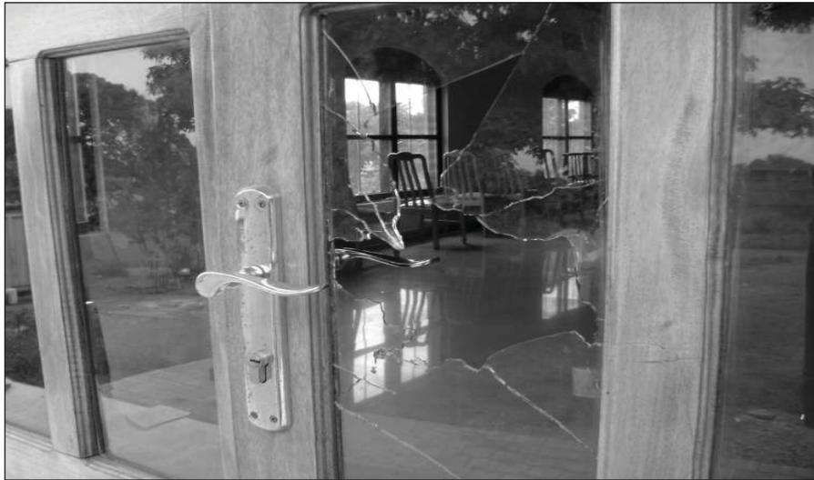
**Figure 1. The bullet hit the glass of the main entrance door.**
